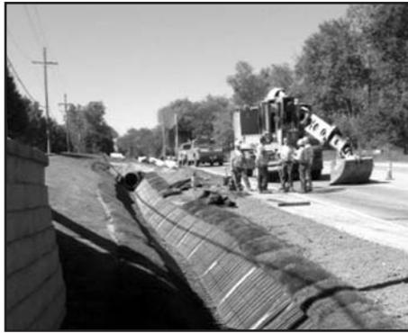
*The RCOC crew installing the smart ditch along Tienken Road in Rochester Hills.*
