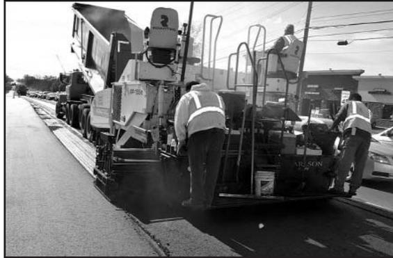
*RCOC's contractor, Pavex, works on one of the spot resurfacing locations. The work includes removing old pavement.*
