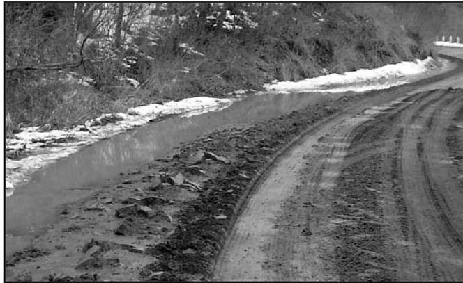
*This is an example of a gravel road where the water is not draining because the ground remains frozen.*
