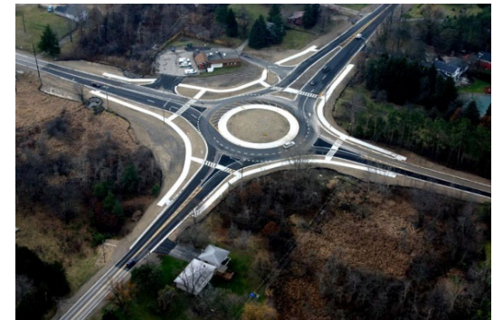
Baldwin/Indianwood/Coats Roundabout in Orion Twp.
