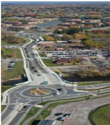
Cover Picture: Dequindre/Avon Road
