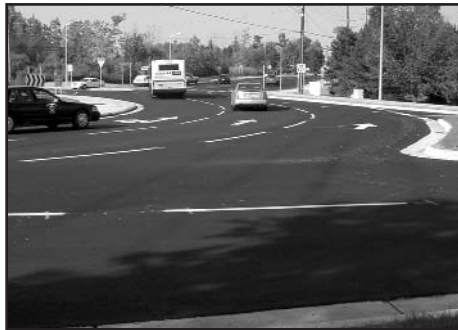
Aerial and ground-level photos of the Maple/Drake roundabout.
