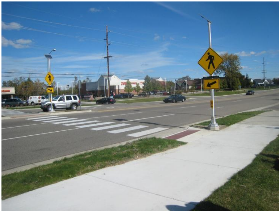
Figure 53: View of Three-Lane Exit Maple Rd. at Maple at Farmington Roundabout, After RRFB Installation
