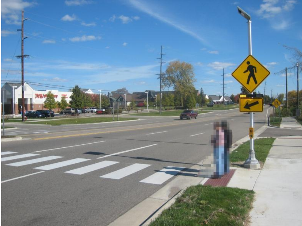
Figure 54: View of RRFB Flashing at Exit Leg Maple Rd. at Maple at Farmington Roundabout
