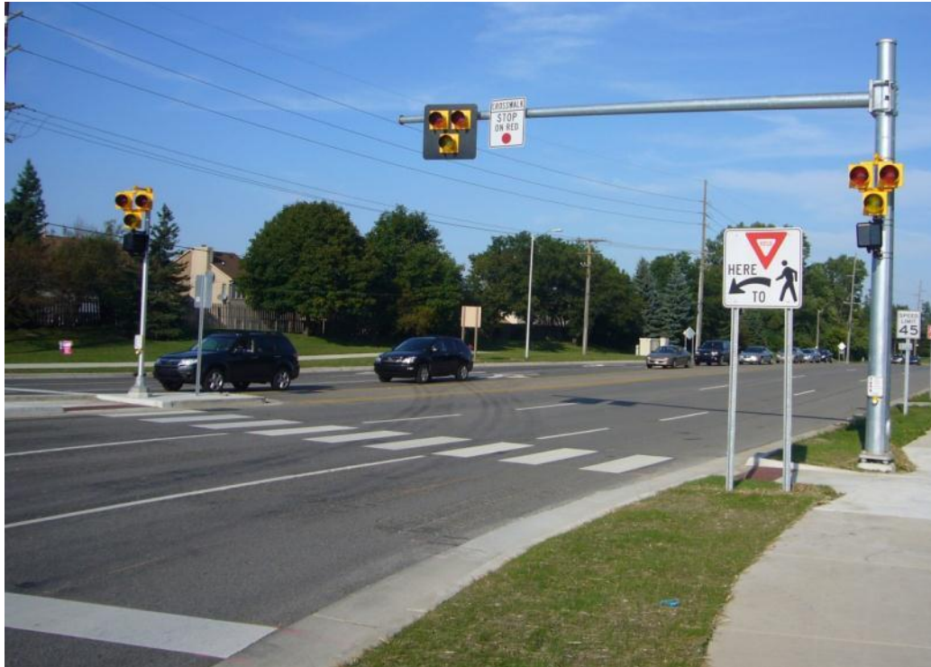
Figure 40: View of Maple Rd Three-Lane Exit at Maple at Drake Roundabout, After PHB Installation
