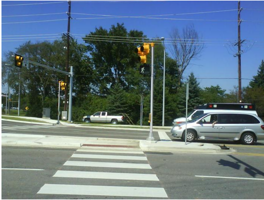
Figure 38: View of Three-Lane Entry and Exit Legs at Maple Rd. at Maple at Drake Roundabout. After PHB Installation and Crosswalk Relocation (Zigzag) at Exit Leg
