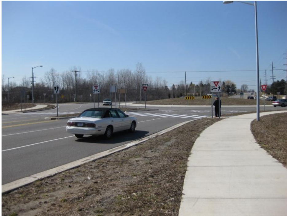
Figure 34. View of Three-Lane Entry and Exit legs Maple Rd. Maple at Drake Roundabout, Before Installation of PHB
