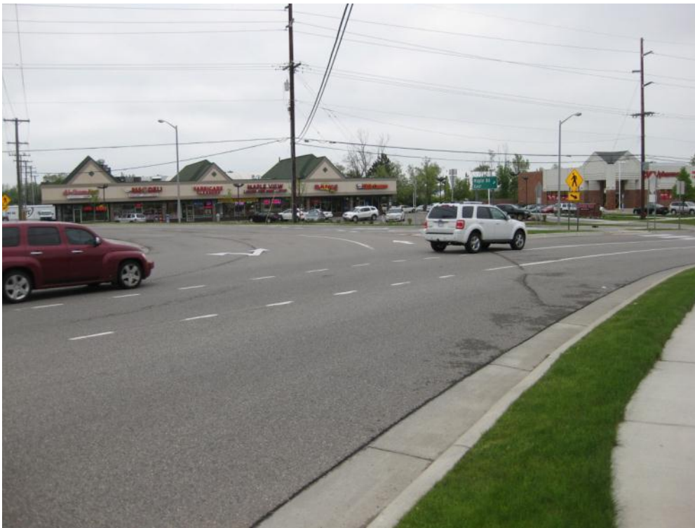
Figure 47: View of Three-Lane Circulating Lanes and Three-Lane Exit leg Maple Rd. at Maple at Farmington Roundabout, Before Case
