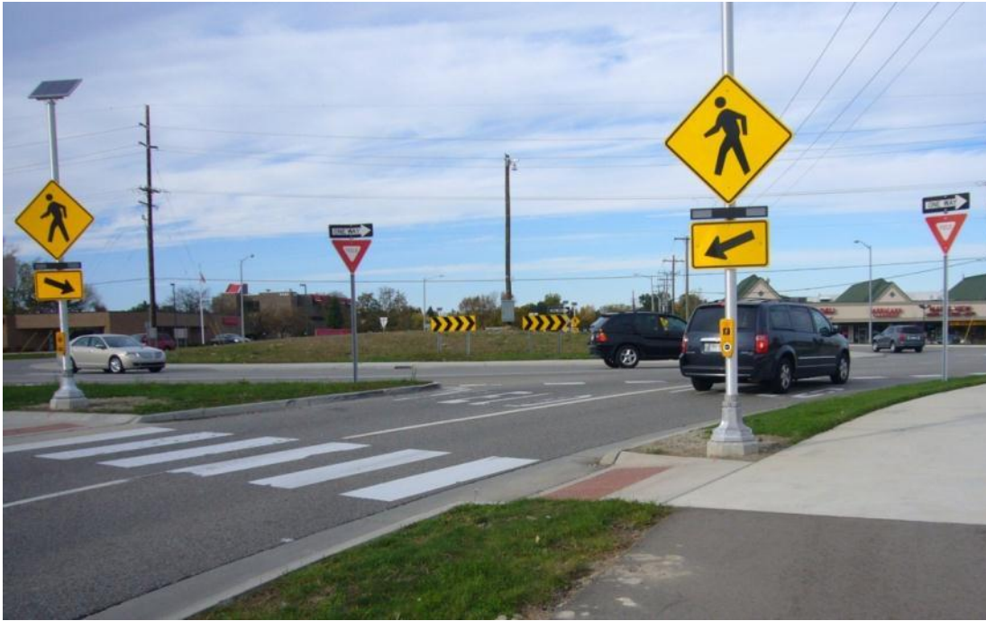
Figure 52: View of Tow-Lane Entry Farmington Rd. at Maple at Farmington Roundabout, After RRFB Installation
