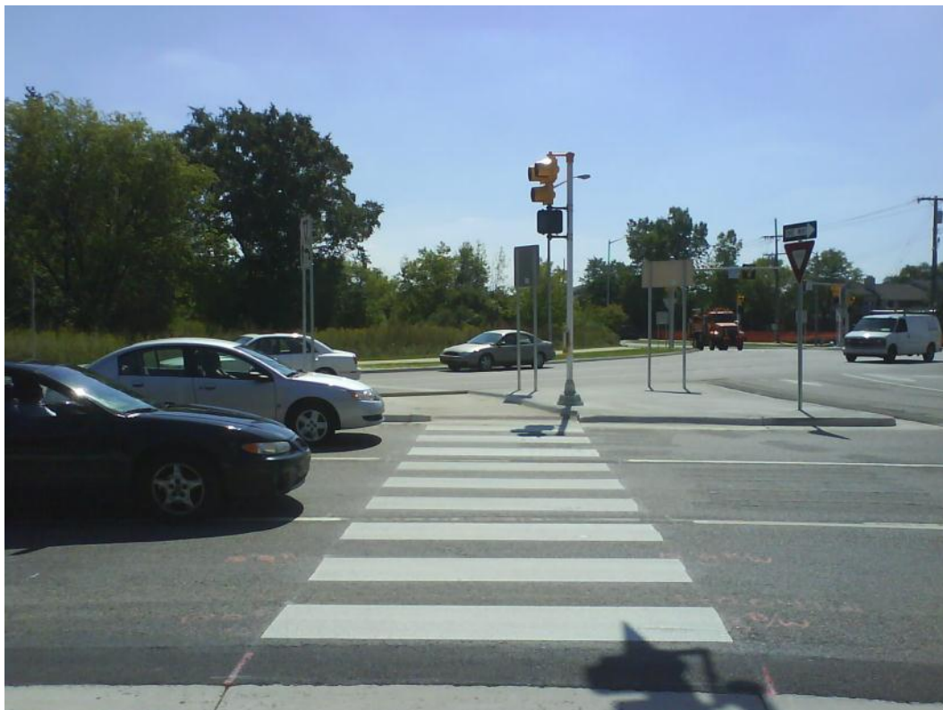
Figure 41: View of Three-Lane Entry at Maple Rd. with Two-Stage Pedestrian Crossing, Maple at Drake Roundabout After PHB Installation
