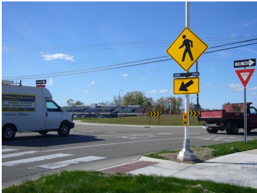
Figure 55: Close-up View of RRFB installed at Entry leg of Maple Rd. at Maple at Farmington Roundabout
