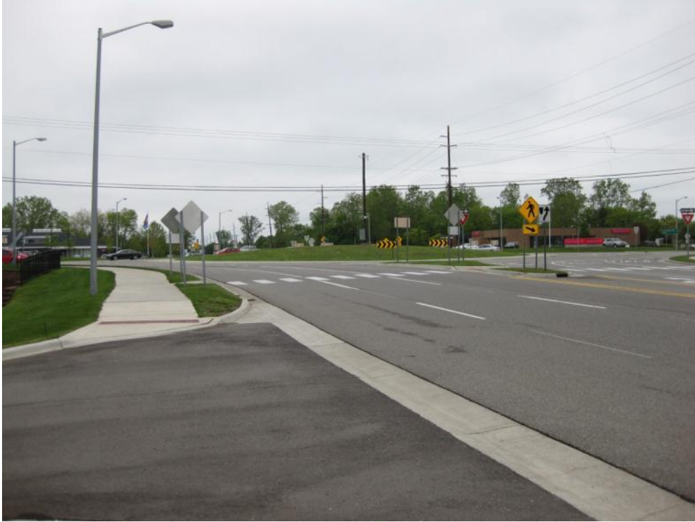
Figure 46: View of Three-Lane Exit Maple Rd. at Maple at Farmington Roundabout, Before Case
