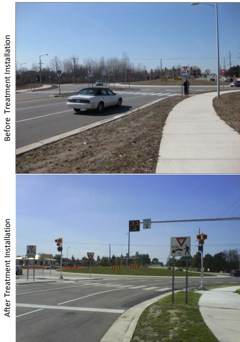
Figure 7: Pretest and Posttest Photos of PHB Treatments at Maple and Drake Roundabout
