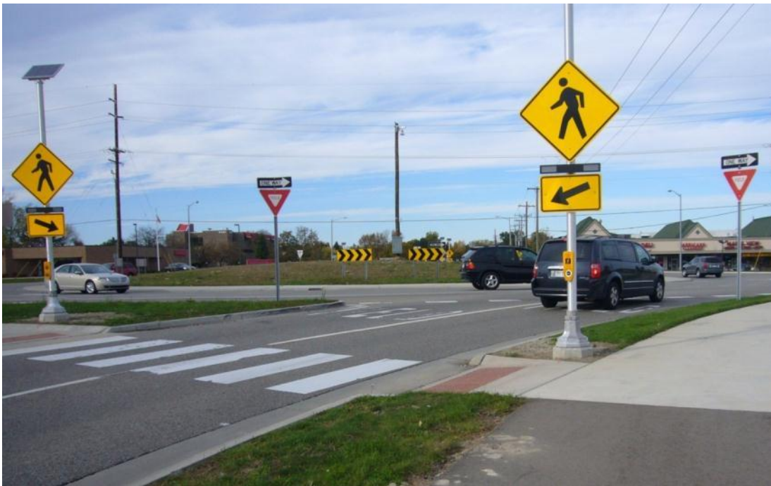
Figure 9: Photo of the RRFB Installation at the Maple/Farmington Three-Lane Entry
