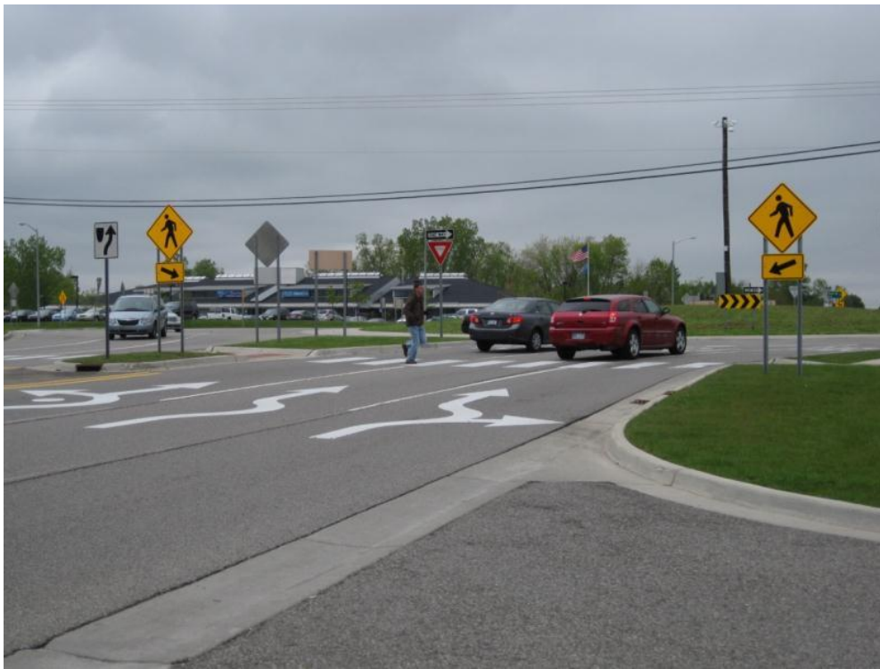
Figure 45: View of Three-Lane Entry Maple Rd. at Maple at Farmington Roundabout, Before Case
