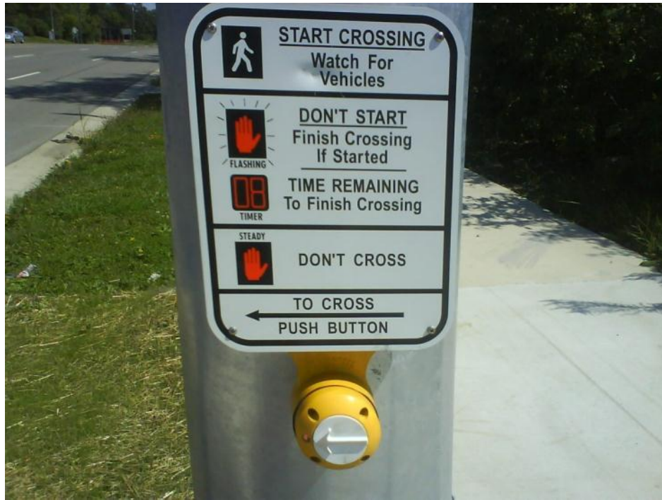
Figure 42: View of PHB (Audible) Accessible Pedestrian Pushbutton at Maple at Drake Roundabout, After PHB Installation
